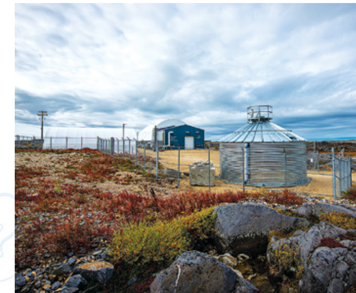
PREVIOUS PAGE: Churchill Marine Observatory located on Cape Merry Road, Churchill, Manitoba
